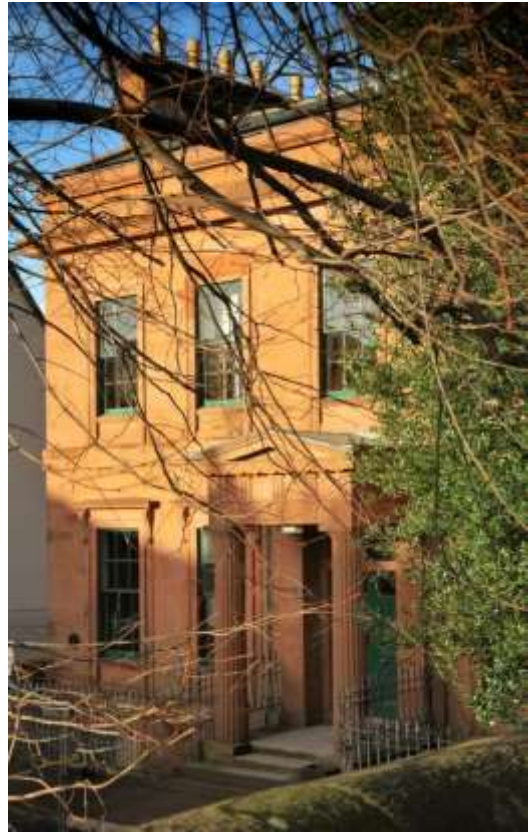
Moat Brae House, Dumfries
